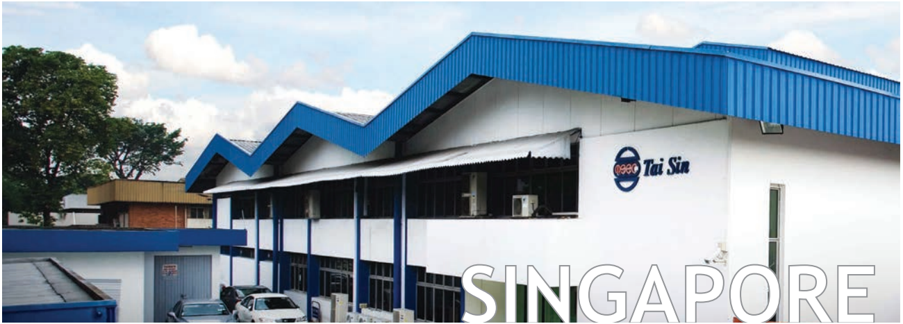
TAI SIN ELECTRIC LIMITED
