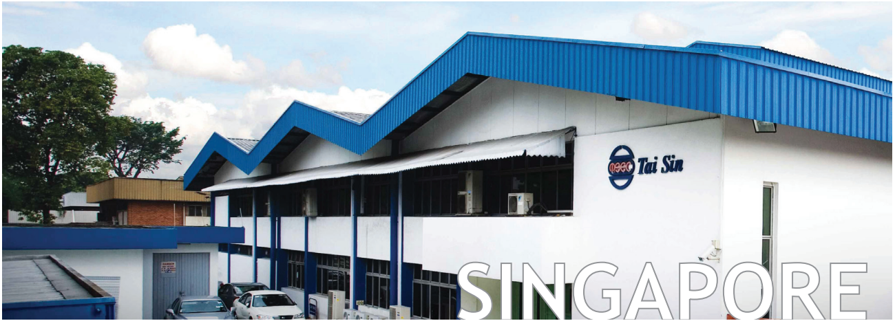
TAI SIN ELECTRIC LIMITED
